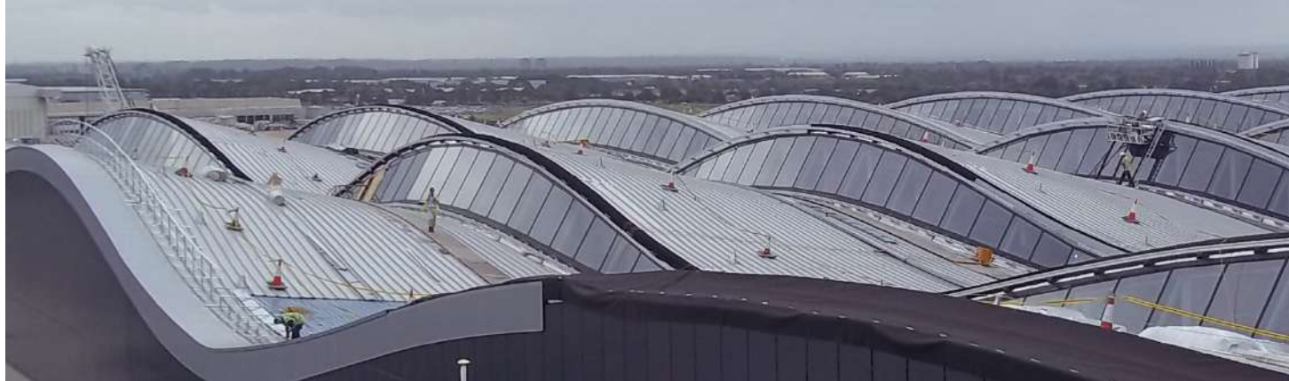
Construction of the new Heathrow Airport terminal (T2A Terminal)
